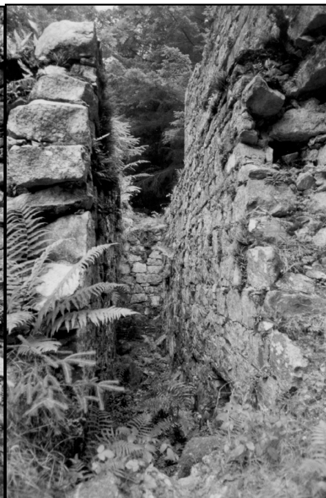
Below middle: Old Crusher House. View from inside showing fixing bolts for the wheel bearing set in the East wall
