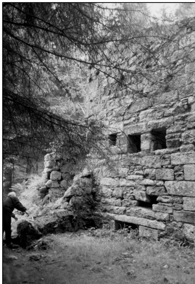
Above: East wall of New Crusher House with the remains of the wheel pit in front
