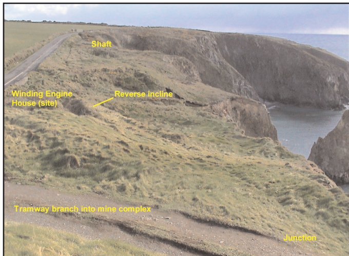
Figure 48. View looking down on the junction, showing the reverse incline extending down slope, and the mine branch passing along the trackway in the foreground.
