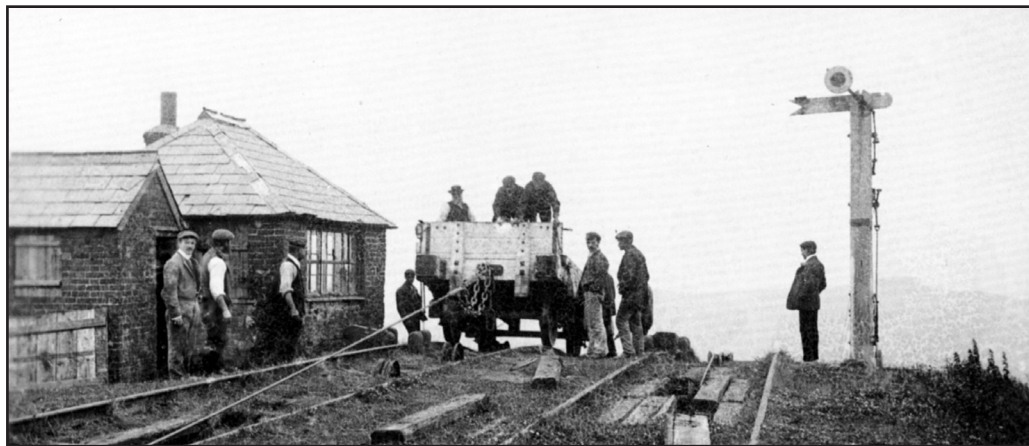
Figure 54. A photograph dated July 21, 1907, showing the configuration of surface infrastructure at the crest of the standard gauge West Somerset Mineral Railway incline, England. Note the Engineman's control hut located at the crest of the incline, and winding ropes passing through slots between each pair of rails on to winding drums mounted below surface. For discussion, see text. Image reproduced by permission of the Dovecote Press.
