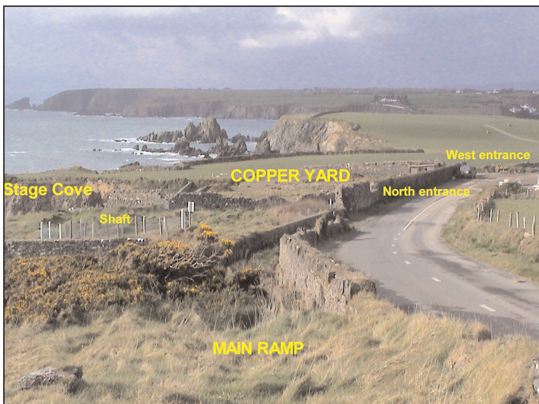
Figure 14. A view looking west across the remains of the Copper Yard.
