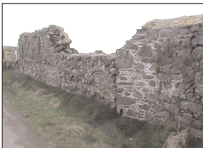
Figure 18. Close up view of the North entrance.
