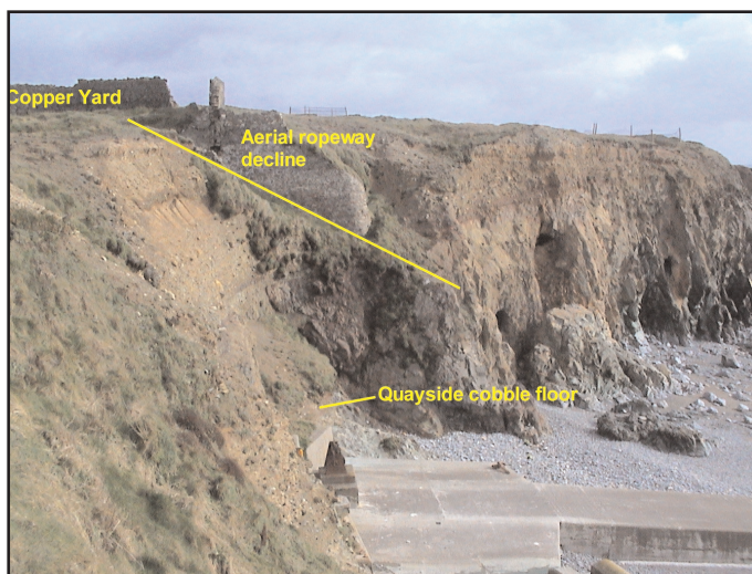
Figure 28. A view looking east along the modern slip way lane into Stage Cove, showing a profile view of the inclination of the aerial ropeway decline from the Copper Yard into Stage Cove.
