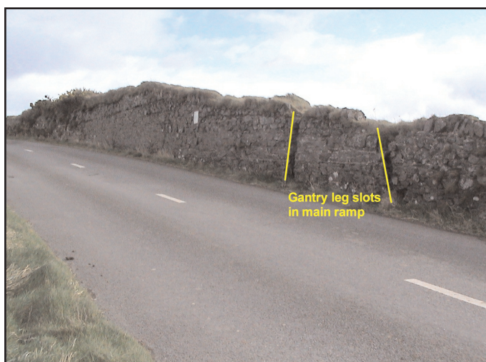
Figure 36. A close up view of the road side edge of the main ramp, the wall top contour clearly reflecting the incline and level sections of the structure. Note the two very prominent near vertical grooves built into the ramp masonry.
