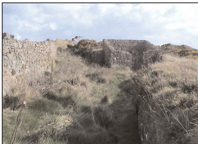
Figure 33. Close up view of roofless shed at base of, and looking directly up the main ramp incline.
