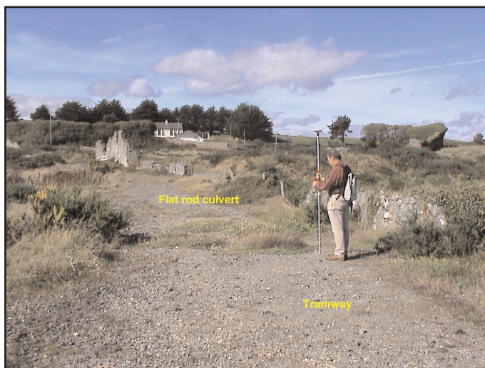
Figure 12. View looking north along the course of the tramway into the Dressing Floor area. Note the location of a flat rod culvert which passes under the tramway.
