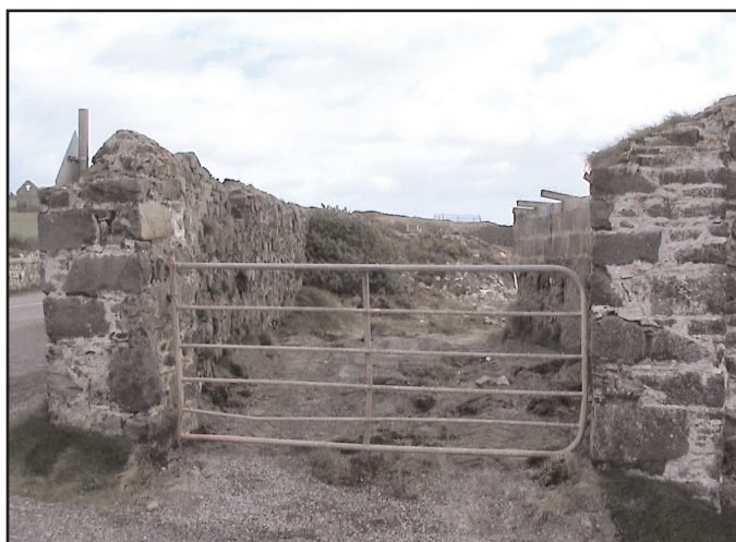
Figure 19. Close up view of the West entrance (at the north-west end of the Copper Yard in Fig. 15).
