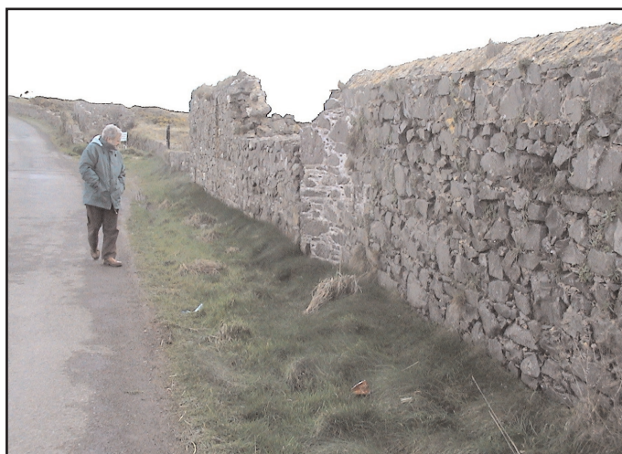
Figure 16. View looking east along the edge of the Copper Yard, with Des Cowman standing on the course of the tramway. Note the very distinct outward curve of the curtain wall at the North entrance (beside the horse whim in Fig. 15), the distinct off-white coloured lime mortar therein contrasting with the darker grey mortar in the near part of the wall, which is constructed entirely of basaltic andesite.
