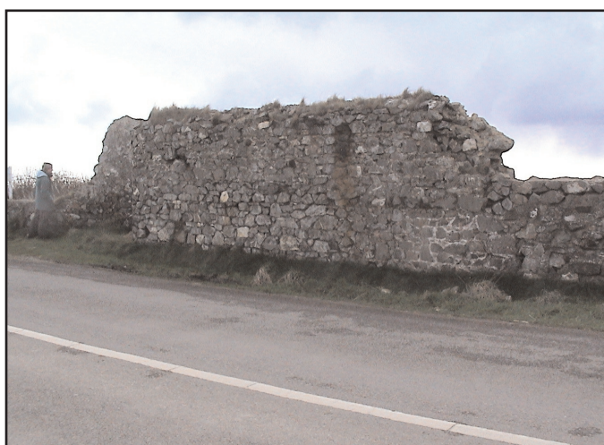
Figure 17. View of wall section east of the North entrance constructed of a very mixed assortment of masonry (andesite, quartz, "Old Red Sandstone" conglomerate) and bricks.
