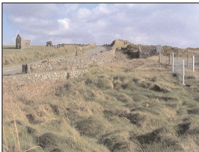
Figure 35. Panorama view looking directly up the main ramp incline, showing the roofless shed on the right hand side, and, on the left, across the coast road, the extant ruins of the Winding Engine House and ancillary features erected in 1838.
