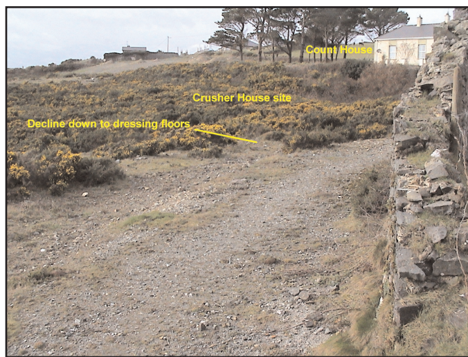
Figure 13. View looking down a shallow incline towards the site of the Crusher House.
