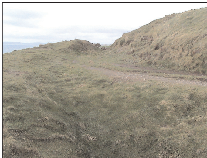
Figure 47. Looking up the top end of the reverse incline, across the junction towards the main tramway incline passing through the shallow rock cutting also visible in Figs. 44, 46.
