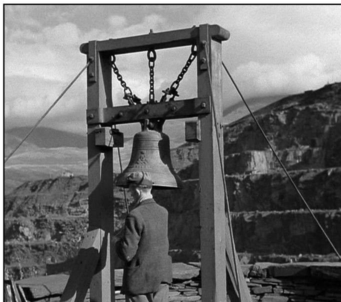
Figure 8. The large bell used to warn of impending blasting at the world's largest slate quarry, Penrhyn, near Bethesda, Wales, shown here in the 1940s. Photograph, British Pathé Films.
