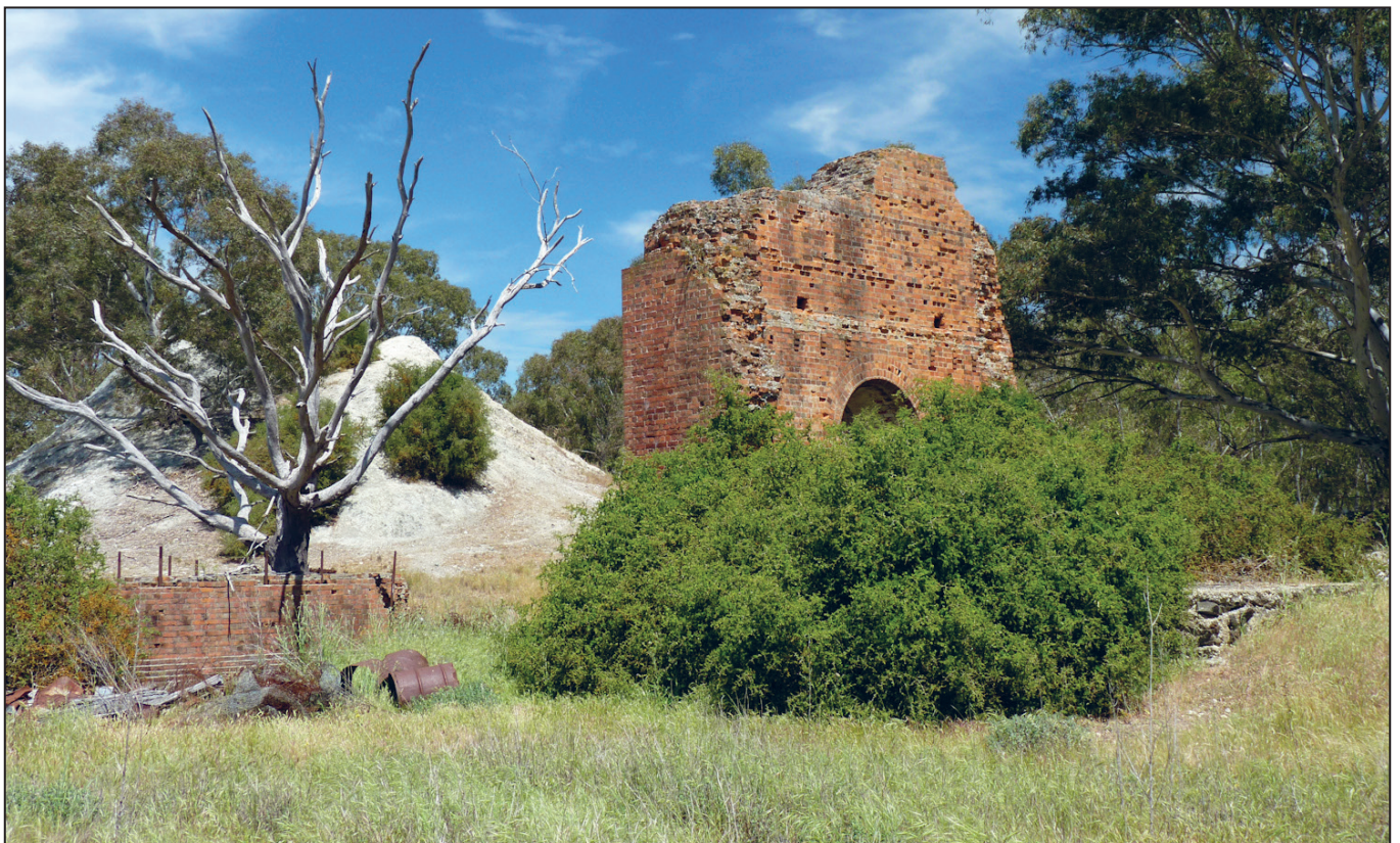
Figure 22. The brick built bob wall of Chalk's No. 1 engine house near Carisbrook
