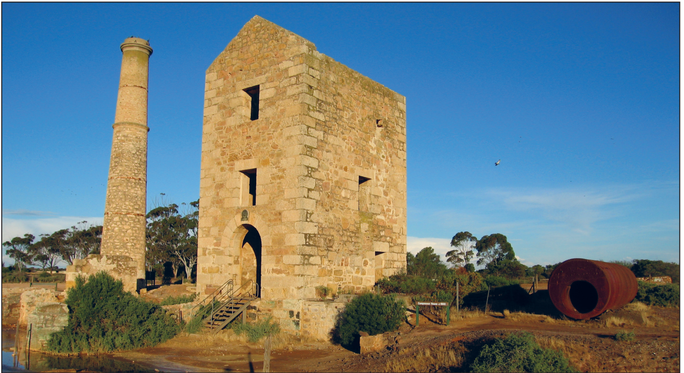
Figure 13. Hughes engine house, Moonta Mines, built for a Harvey's of Hayle engine
