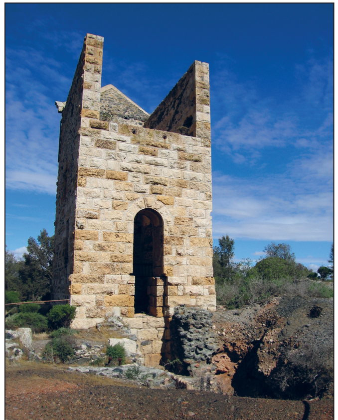
Figure 14. Harvey's engine house, Wallaroo Mines, Kadina
