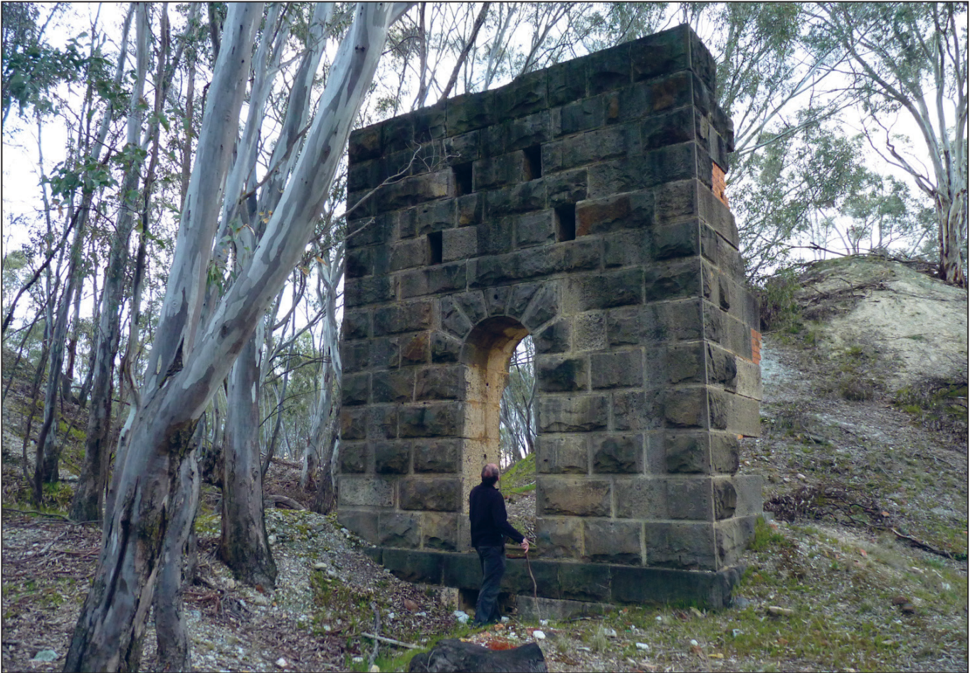
Figure 21. Each block of the stone-built bob wall of the North Duke engine house hidden deep in the bush, bears an engraved number, suggesting that the house, and probably its engine, had been moved from elsewhere
