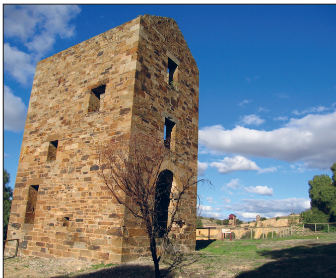
Figure 10. Graves engine house, Burra, built for an 80-inch engine that was never installed
