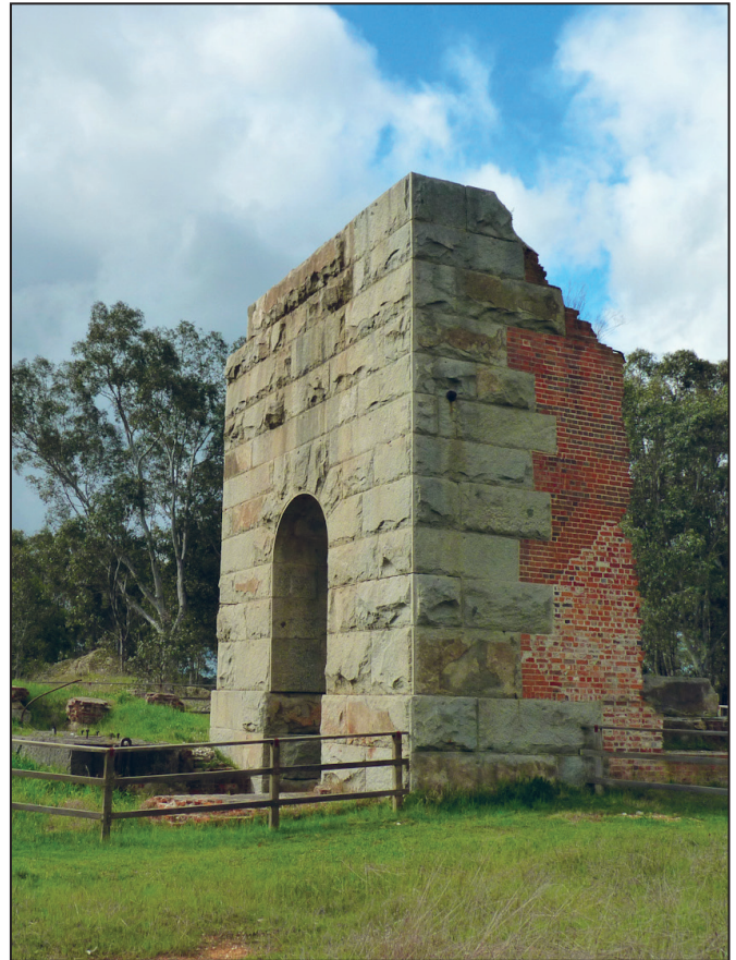
Figure 20. The bob wall of the Grand Duke Engine House, Timor, which accommodated a Harvey's of Hayle engine
