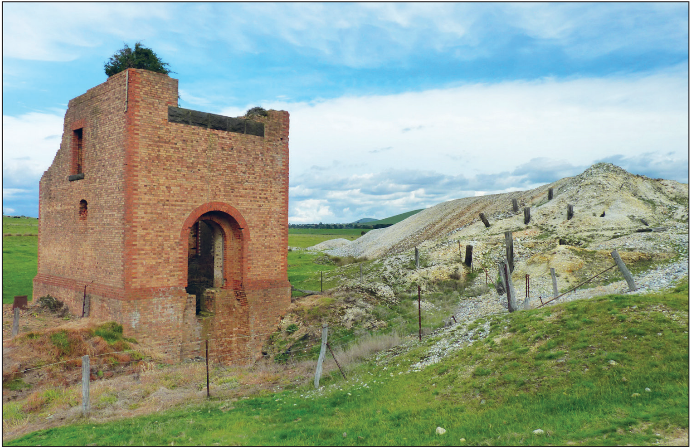
Figure 19. The well-preserved brick built engine house of the Berry No. 1 Mine near Smeaton
