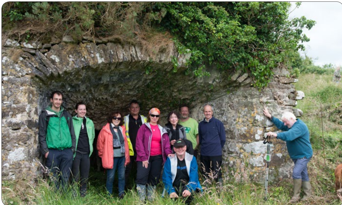
The Derryoover Furnace which Paul and fellow volunteers had pre-cleared of vegetation. There is no upper stone course at the building suggesting it may not ever have been finished
