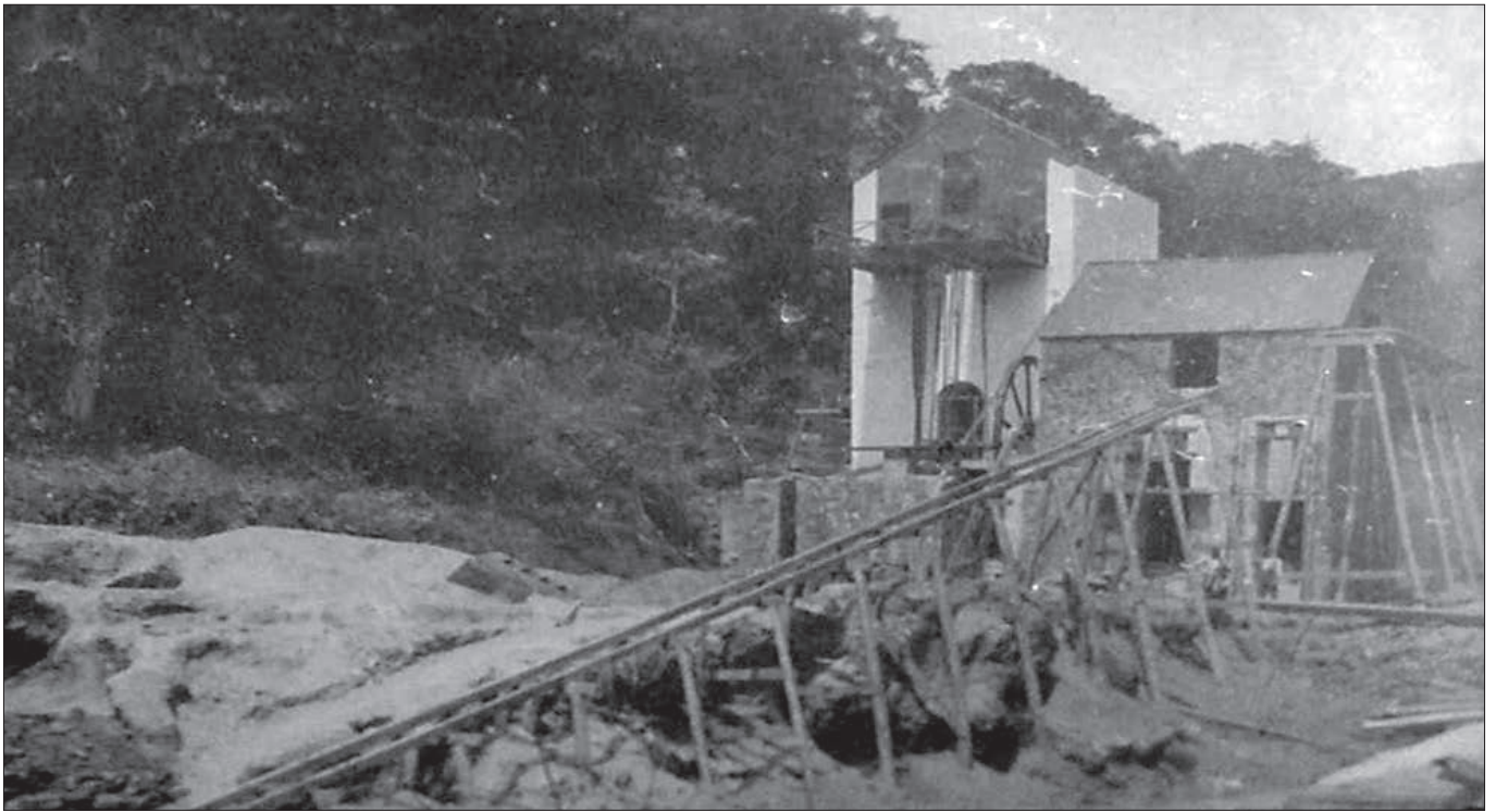
Fig. 2: Cotehele Consols within the Danescombe Valley, Cornwall, c.1880, with the crusher house (right) adjoining its driving beam engine (SX 42298 69369, extant); the feed ramp is clearly evident to the fore and two figures can just be discerned underneath this at the foot of the house. The loading at the front of the driving engine was built to accommodate two flywheels although only one is installed at this date. (EBay web auction listing, accessed: April 2013)
