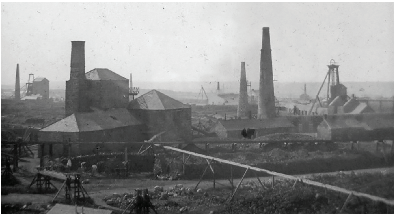
Fig. 3: Another Cornish scene, understood to have been Tincroft Mine within the Central Mining District around the turn of the twentieth century (SW 66791 40823, site of); a combined part time Cornish rolls crusher and whim installation can be seen to the left comprising engine house and chimney (to the rear of the group) with the adjoining boiler and crusher houses to the front left and right, respectively. The crusher feed ramp can just be discerned to the right and in front of the crusher house. The image is also interesting in that it shows a supporting gantry and dolly wheel frame (bottom left) which was used to facilitate remote haulage from a nearby shaft and to keep the haulage cables clear of the mine road. (EBay web auction listing, accessed: April 2013)
