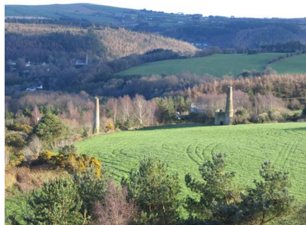
Looking over Ballygahan engine houses to Avoca.
