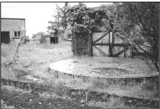
Figure 8. View of circular shaft, capped with concrete in 1988. Behind is the shaft signalling and access shed, and to the left, part of the electrical-mechanical workshop.
