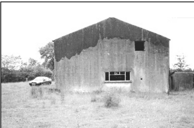
Figure 7. View of former hoist house. Opening at upper right of wall allowed for passage of pulley cables to head-frame.
