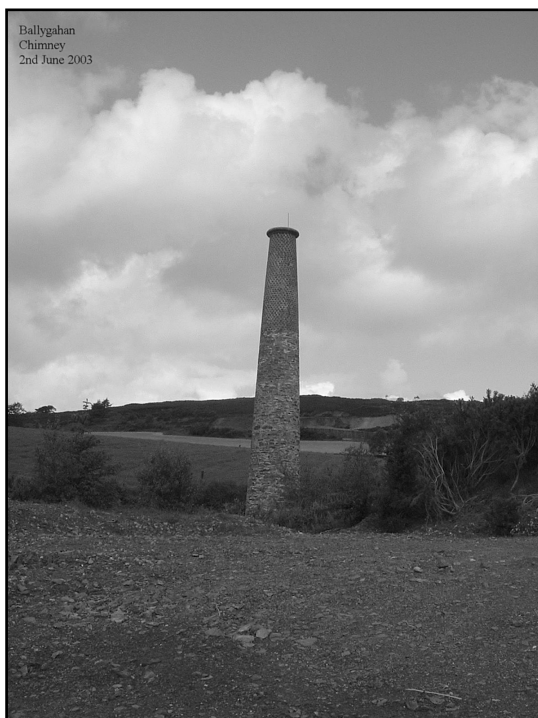
Figure 7. The engine house chimney at Ballygahan.
