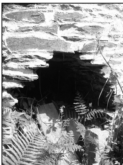
Figure 8. The base of the chimney.
