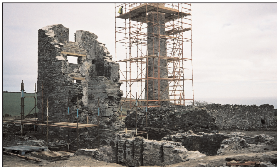
Figure 16. The winding engine-house at Tankardstown. The vertical grooves in the wall in the foreground are for the long retaining bolts that secured the winding drum. The higher wall between the engine-house and the chimney beyond it is the long wall of the adjoining boiler-house.
