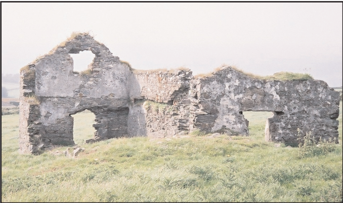
Figure 10. Ruined engine-house, Stage Cove.
