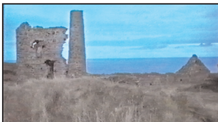
Figure 10. Chimney stack conservation and reconstruction: above, as visible in the 1970 film, "The McKenzie Break" (reproduced by permission of MGM Films); right, similar view, 2004. Note and compare the loss of part of the Winding Engine house wing wall between 1970 and 2004, and also the external winding drum pit on the nearside of the building, with prominent grooves for axle hold down bolts; far right, during reconstruction of the brick chimney top in 2005.
