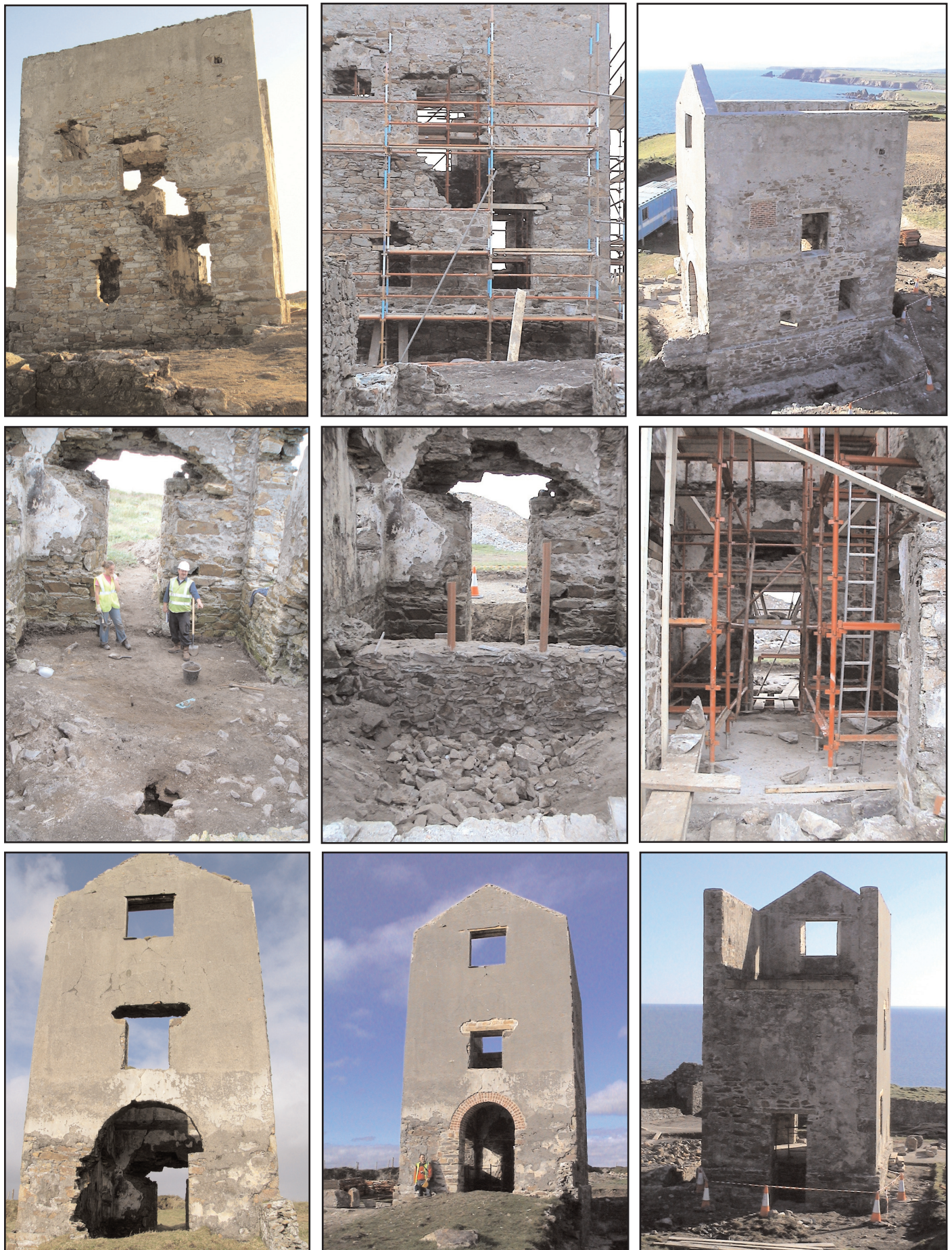
Figure 7 Bottom row: views of rear gable and bob walls: before and after conservation works on gable wall (left, centre: note reconstructed masonry and brick arch over cylinder doorway, and replaced oak lintels in windows above); and after completion of works on Bob wall (compare with views in Figs. 3 and 6 before conservation works).
