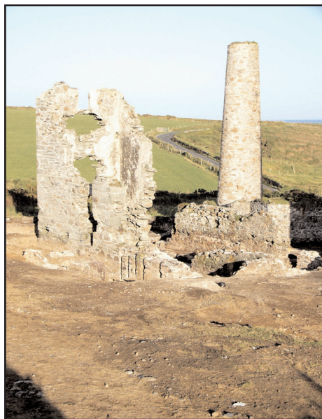
Figure 10. Chimney stack conservation and reconstruction: above, as visible in the 1970 film, "The McKenzie Break" (reproduced by permission of MGM Films); right, similar view, 2004. Note and compare the loss of part of the Winding Engine house wing wall between 1970 and 2004, and also the external winding drum pit on the nearside of the building, with prominent grooves for axle hold down bolts; far right, during reconstruction of the brick chimney top in 2005.
