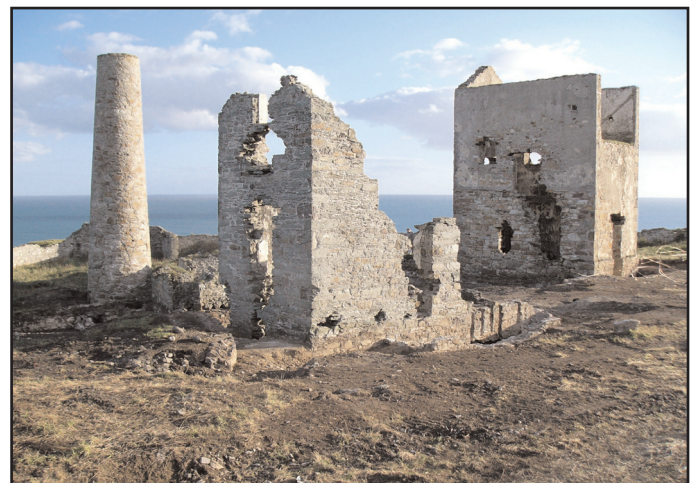
Figure 3. Tankardstown Engine House complex, September 2004, after completion of archaeological excavations, prior to conservation works. Pumping Engine house on right, winding engine house centre, and single chimney which served both boiler houses on the left.
