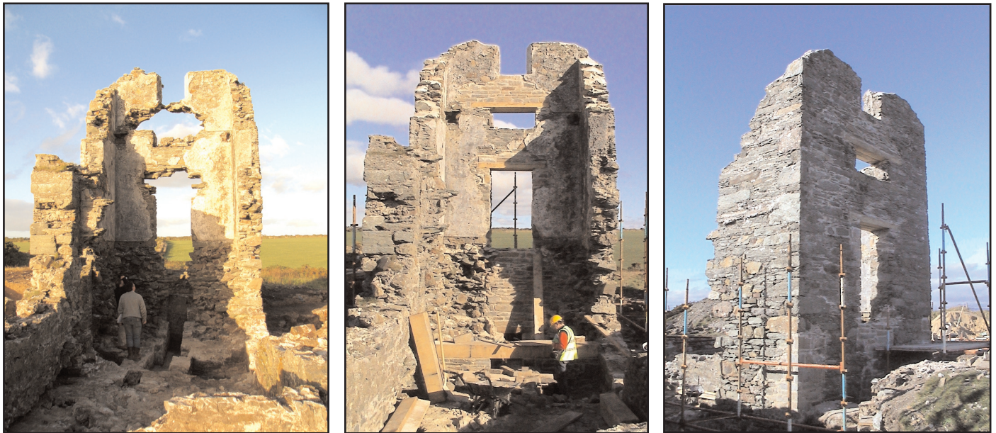
Figure 9: Above left - Tankardstown Winding Engine House, viewed from the same perspective as Fig. 8b. The original cylinder floor level was located just below the base of the internal plaster level visible above the people standing in the area of the completely robbed out cylinder bedstone masonry plinth. Note the crow hole tunnel and drainage channel located beneath the plinth. Part of internal bob beam support wall visible on right (the isolated pillar in Fig. 3). Flywheel and crank originally located along inside edge of left hand side wing wall (left foreground), and to external winding drums outside the building, on the left.
