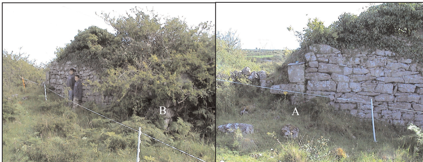
Figure 9. Building gable wall section, infilling between two remnant wall sections constructed of very finely dressed limestone: Pillar A, on the left, east side; Pillar B on the right, west side, and partially obscured by bushes.
