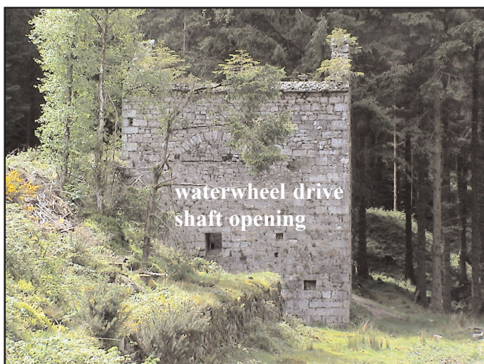
Figure 14. A view of the New Crusher House, looking west northwest. Note the prominent square opening for the drive shaft from the waterwheel (located in a slot parallel to the east facing wall visible: Figure 16) to the ore crushing machinery, which was housed inside the building. Compare with plan and section views shown in Figure 15.
