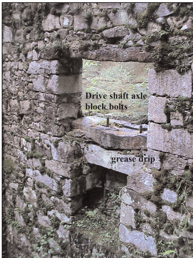
Figure 23. Drive shaft axle block bolts
