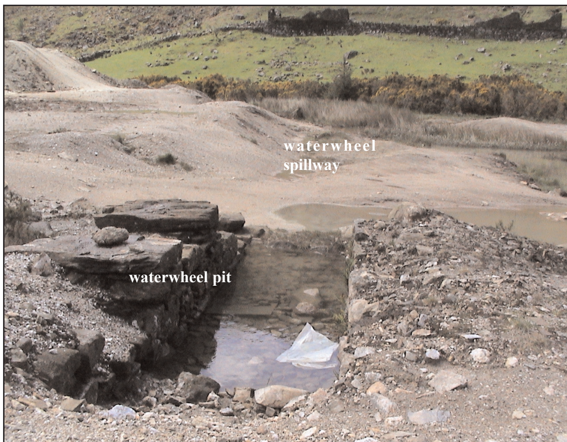
Figure 6. Waterwheel pit, with presumed axle bearing blocks at the top of the low wall on the left; and the presumed course of the spillway marked by a linear depression in the area beyond. Note the building ruins in the background, on the opposite side of the Avonbeg river.
