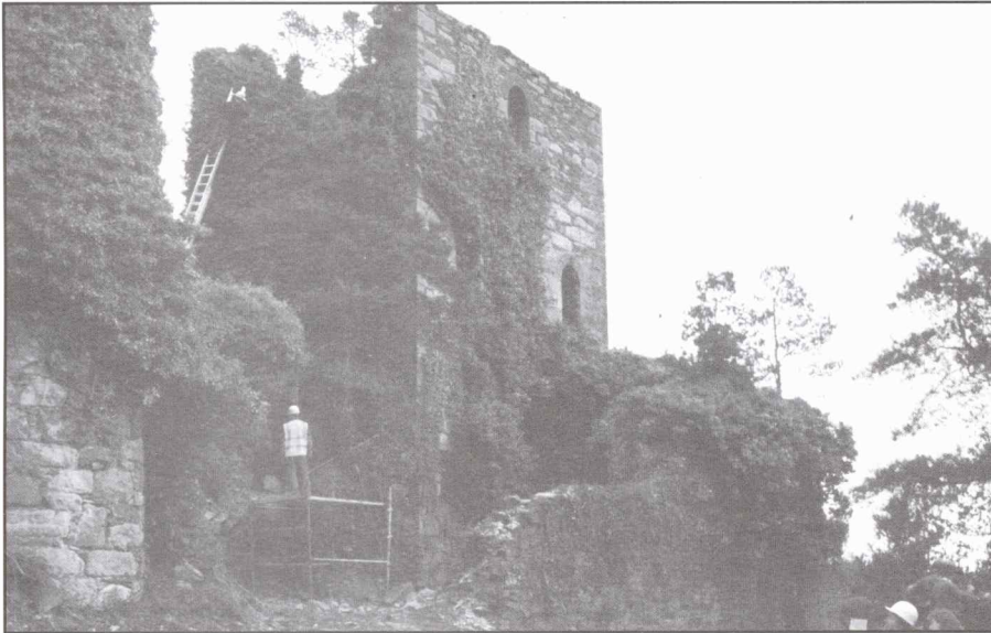
Figure 4. General view of the house and stack from the north. The rear bob opening is obscured by ivy. The author at the top of a ladder checking out the location of the back bob amidst the ivy, October 1997. (Roz Cundick)
